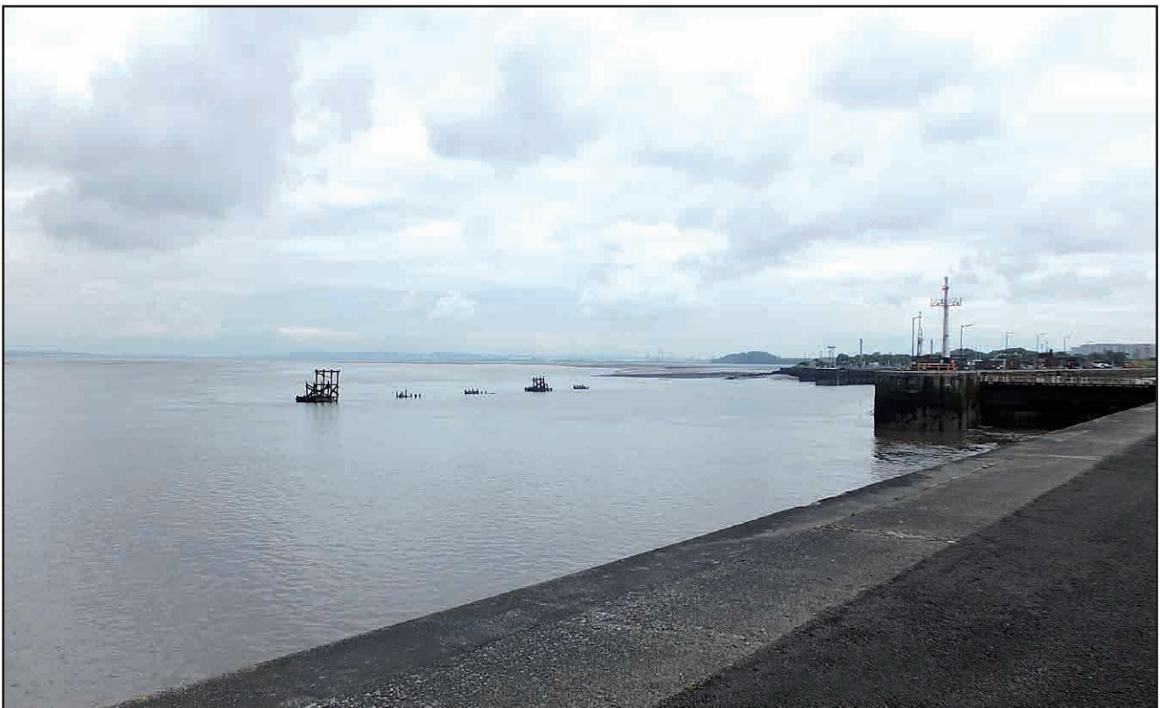
Figure 1: View of exposed dolphins
